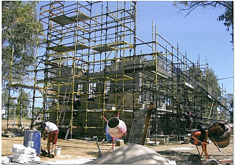
Construction underway on the Carriage House
